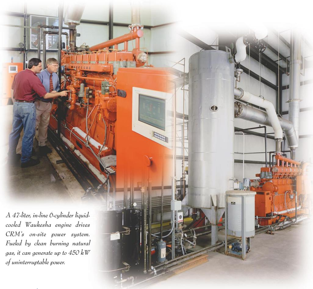
*A 47-liter, in-line 6-cylinder liquid-cooled Waukesha engine drives CRM's on-site power system. Fueled by clean burning natural gas, it can generate up to 450 kW of uninterruptable power.*
